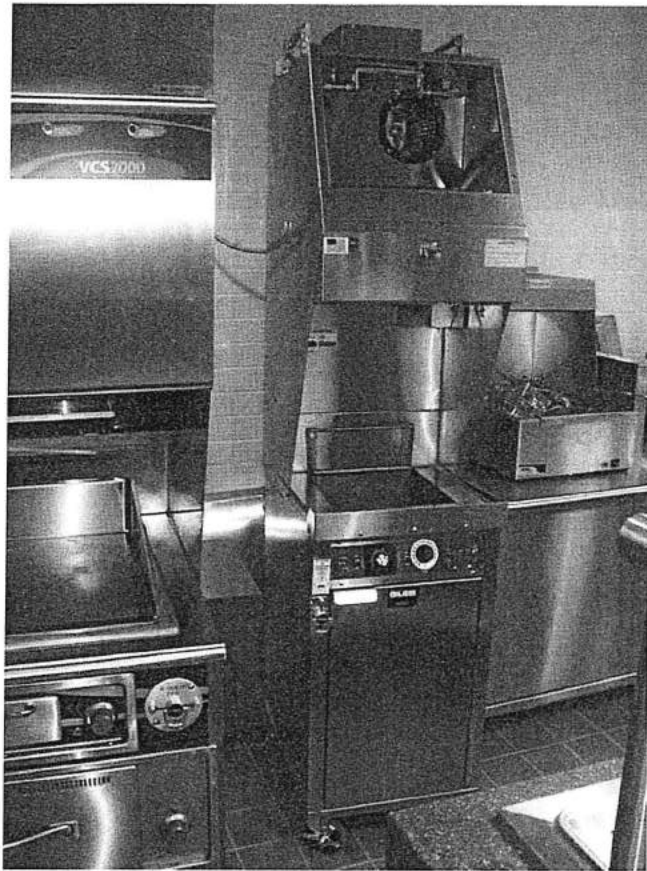
Figure 507.1(2) ELECTRIC DEEP FAT FRYER WITH RECIRCULATING HOOD
